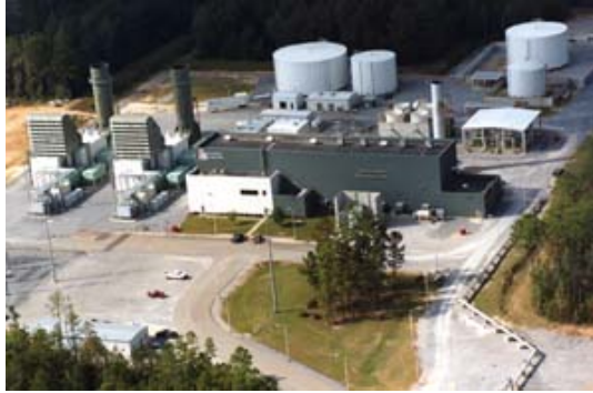
Figure 2.20 Aerial view of McIntosh CAES plant
